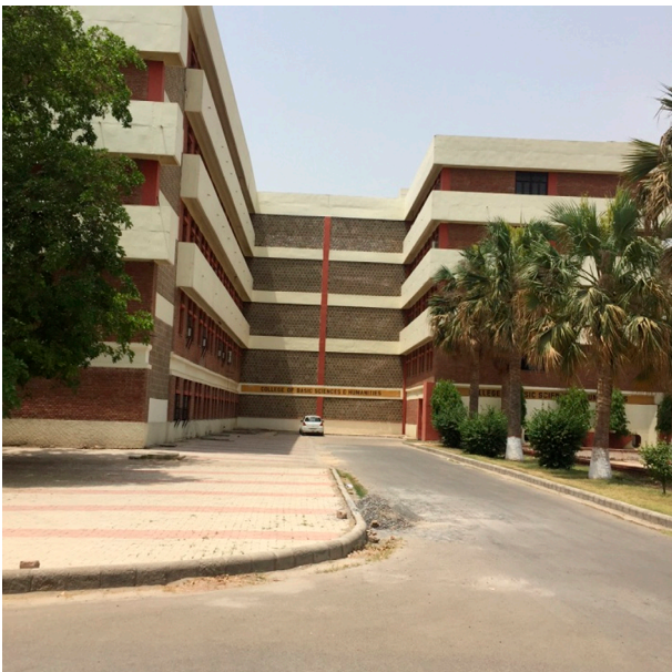
Figure 9. Building of the College of Basic Sciences & Humanities having sun shade projections where A. dorsata made nests. The colony in Figure 3 was present on the projection of this building. On four floors, this building alone carries about 5000 m surface length for about 2500 potential nesting sites.
