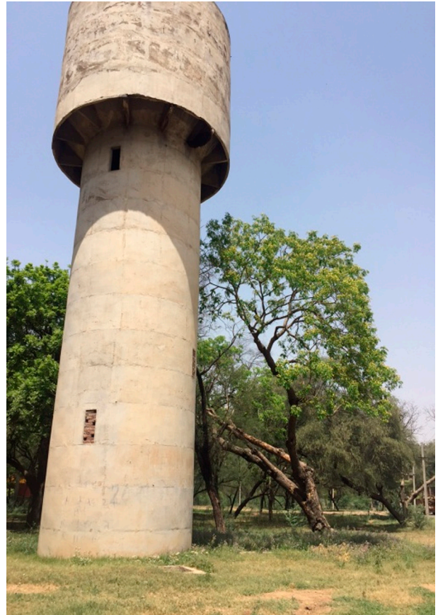
Figure 4. A. dorsata nesting on the water tower building, WT-1 (height of the nesting sites was about 15 m from the ground). Only 5 nesting sites were occupied with different annual occupations whereas remaining 9 sites of this tower and all the 8 sites of another similar tower WT-2 were not occupied even for once during the entire period of this study. The tree adjoining to the tower is siris ( A. lebbek ), an excellent nectar source where this bee was first reported foraging during night time (Sihag, 1984). The angle of all the nesting sites was around 30°.
