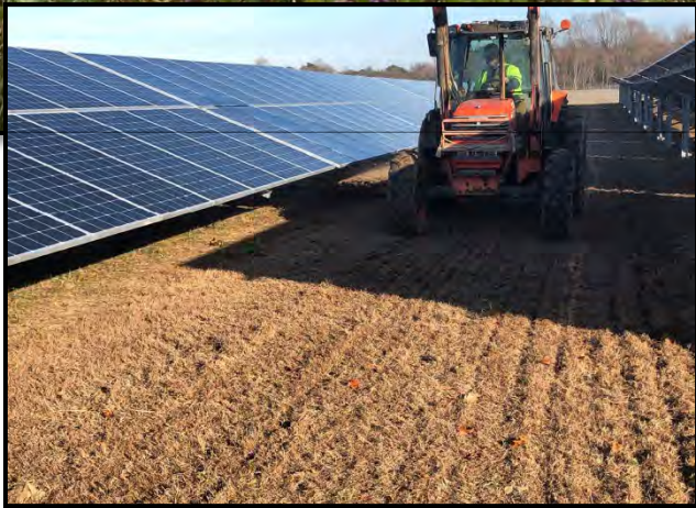
Drill Seeding Between Erected Panels, YES, We Do That!
